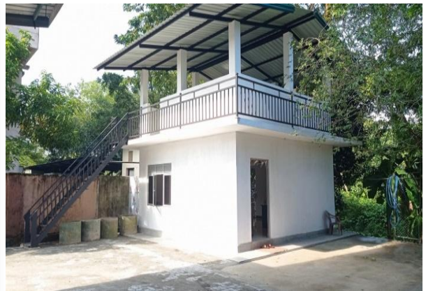
Construction of the driver's lounge at the head office
